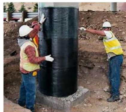
Figure 13. Strengthening of a RC columns with FRPs
